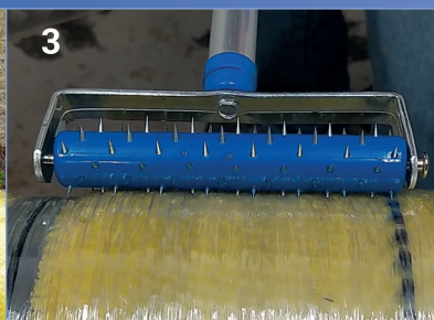
Perforation du film de compression
